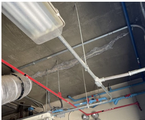
Figure 11: Odor Control Building
