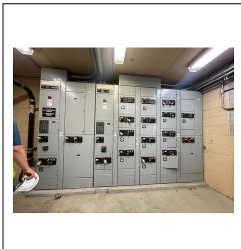
Figure 16: 2009 MCC inside digester 1 room
