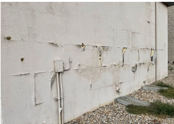
Figure 5: Generator Building 1 Exterior
