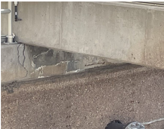
Figure 6: South Train Aeration Basin Concrete
