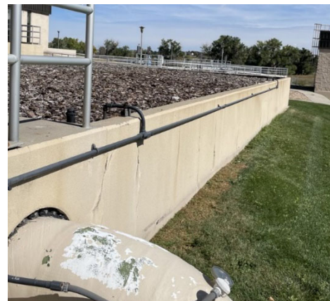
Figure 10: Odor Control Basin
