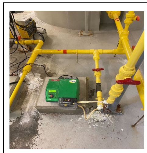
Figure 9: Hypochlorite corrosion.
