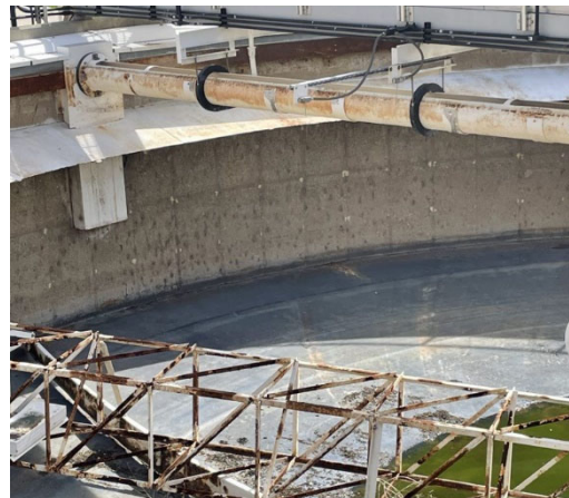
Figure 7: South Train Secondary Clarifier Mechanism and Concrete
