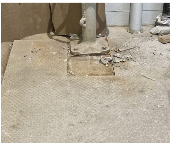
Figure 4: Old Headworks Concrete
